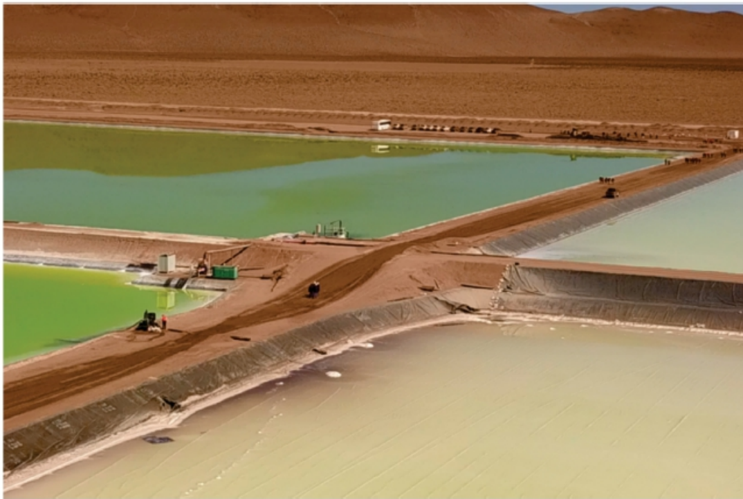
Figure 14.4 Evaporation Ponds – Close Up
