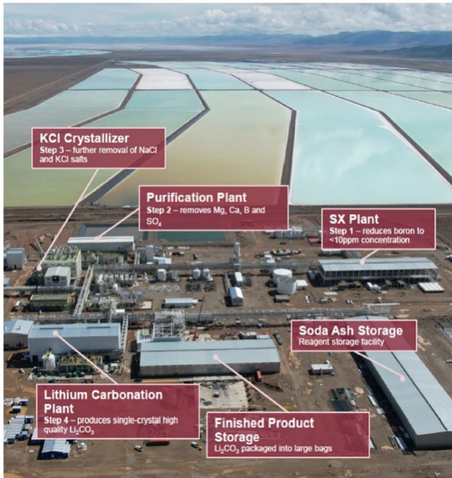
Figure 15.1 Aerial View - Main Facilities
