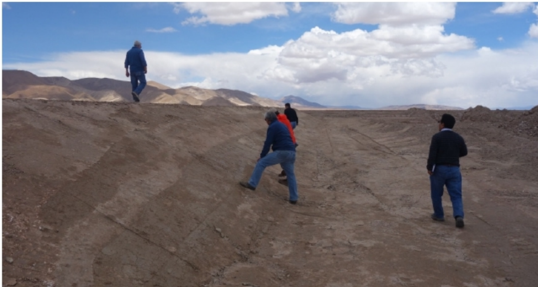
Figure 14.3 Testing of Berm Material
